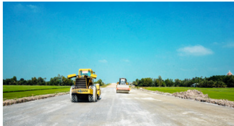
Lo Te – Rach Soi - Embankment construction
