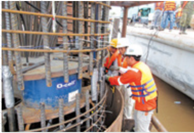
Cao Lanh Bridge - O-Cell load test for bored pile with diameter of 2500mm
