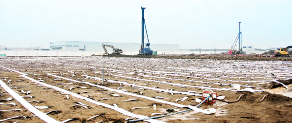
LG Display Vietnam Hai Phong - Soil improvement by PVD installation & DCM method: 50,234m
