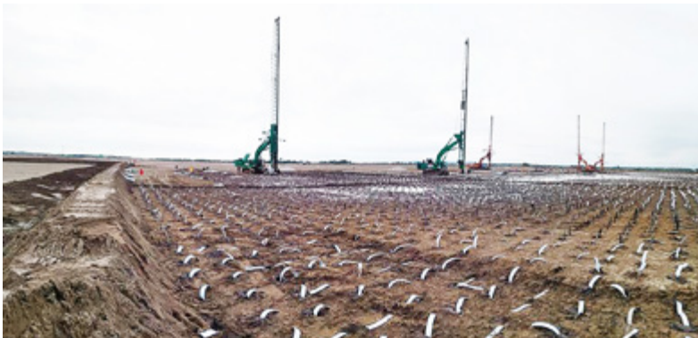
Long Son Oil Refinery Plant (Ba Ria, Vung Tau) - Soil improvement by PVD installation and Vacuum Pre-loading method, Dynamic Compaction
