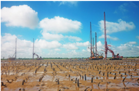
Thilawa Port (Myanmar) expansion - Soil improvement in PVD method
