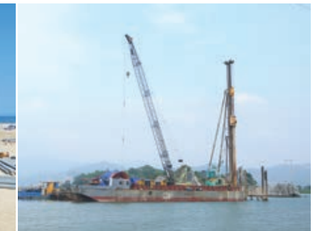
Thi công cọc khoan thả Sobotory Method Execution, Piling with Pre-boring
