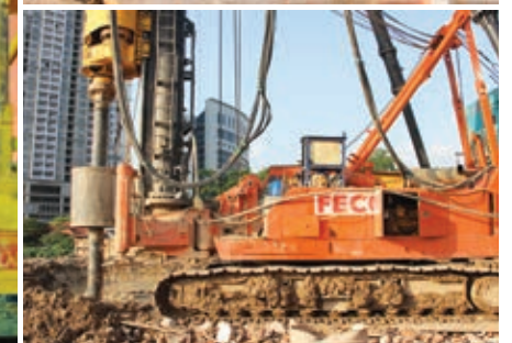
Cọc khoan hạ/ Pile Injection Method
