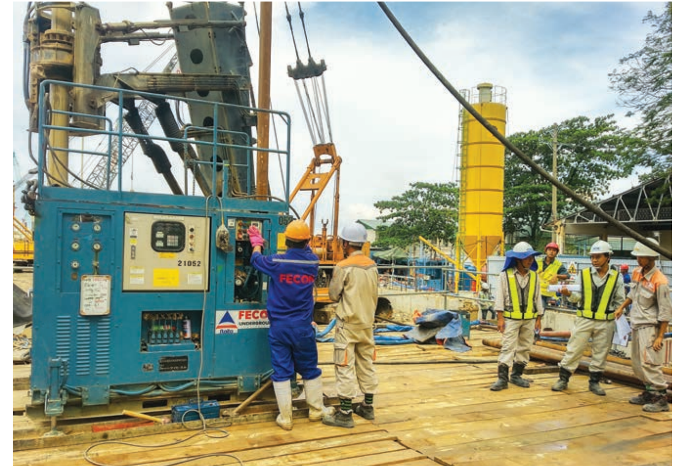
Xử lý nền, chống thấm công trình ngầm bằng các phương pháp Jetgrouting, Chemical Grouting, Tam Grouting Soil improvement, waterproofing of underground structures by Jet Grouting, Chemical Grouting, Tam Grouting
