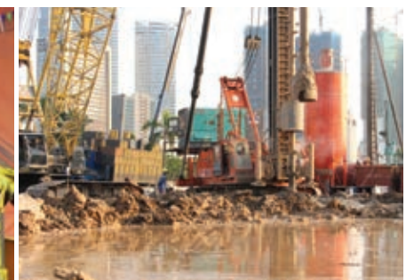
Thi công cọc khoan thả Sobotory Method Execution, Piling with Pre-boring
