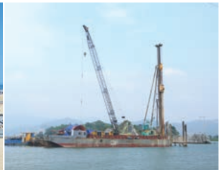
Thi công cọc khoan thả Sobotory Method Execution, Piling with Pre-boring
