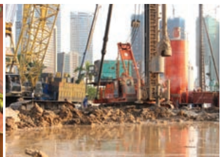
Thi công cọc khoan thả Sobotory Method Execution, Piling with Pre-boring
