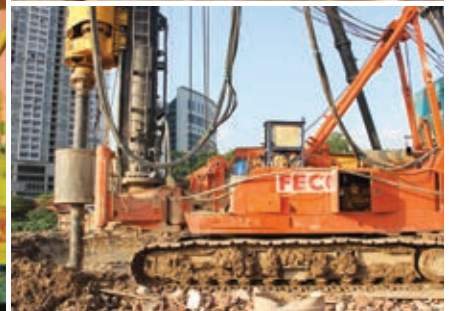
Cọc khoan hạ/ Pile Injection Method
